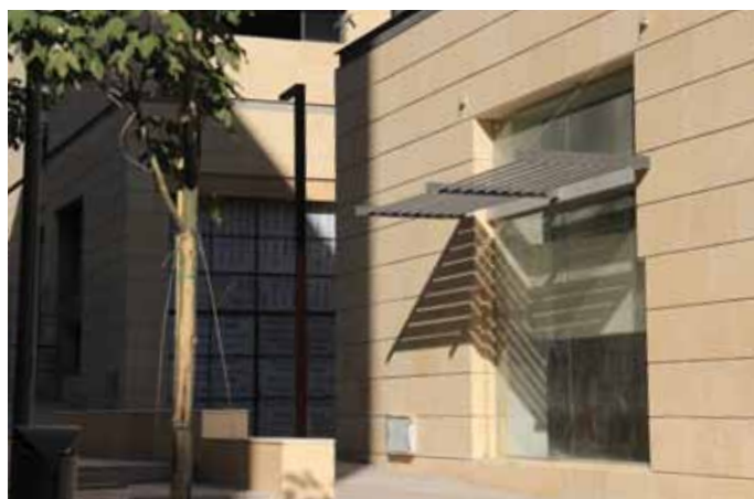
Horizontal window shading in Abdali, Jordan
