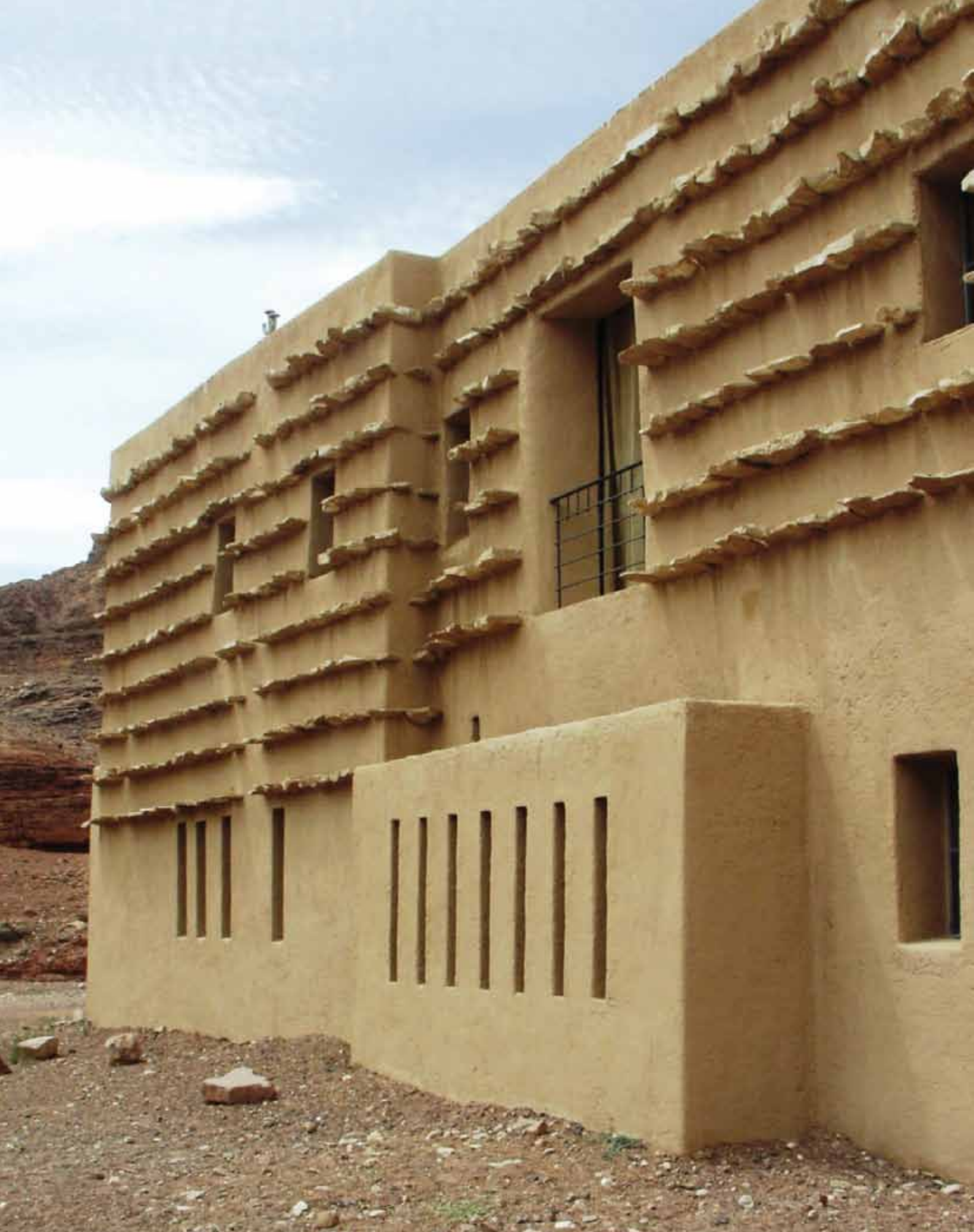
Ecolodge Feynan Jordan. In one of the hottest areas in Jordan, and where there is no electricity connection, this environmental project is developed with the following energy saving measures: court yard building, window design (dimensioning and location) for optimal day lighting and minimum cooling (the interior is designed to make use of candle light as an alternative to electrical lighting), improved thermal resistance for walls and roof, shading for windows and elevation in Yemeni tradition, and solar water heaters. A photo voltaic system covers the electricity demand for food cooling. Architect Ammar Khammash.
