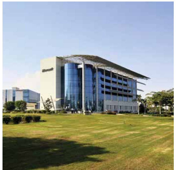
The roof receives the highest solar radiation, shading is a good solution, office building in Giza, Egypt.
