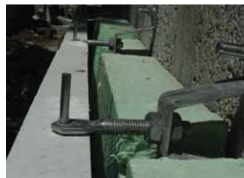
Wall construction, Dutch Embassy, Jordan
