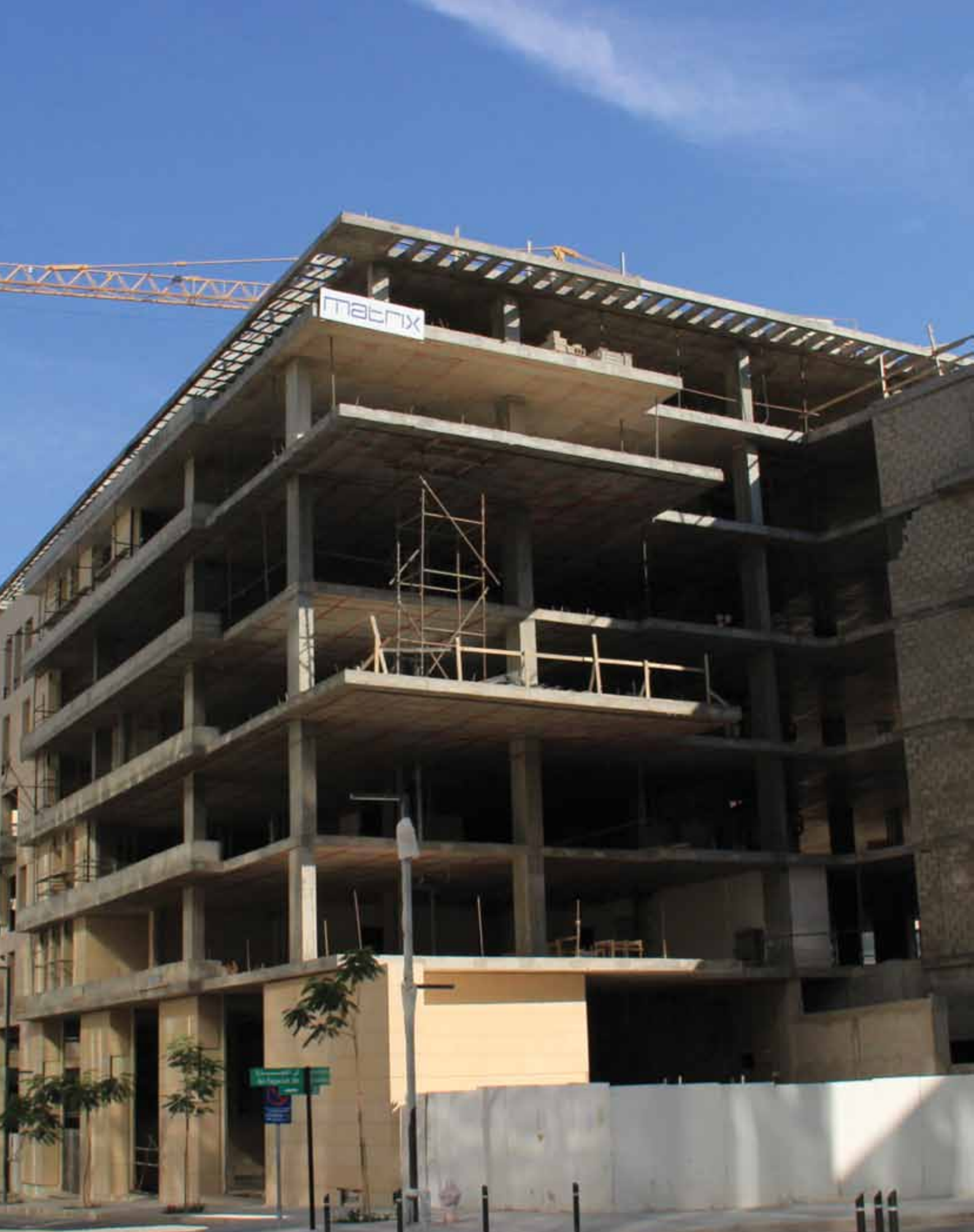
The Crystalle building in Amman, Jordan, here under construction, is designed as a Green Building. It includes the following energy saving measures: insulation on the interior side of walls, (5cm polystyrene and 10cm light weight concrete blocks) and on the roof ( 5cm of polystyrene), windows with double glazing, window frames with thermal break, shading devices, best practice efficient HVAC systems and solar water heaters. Delivery is planned for 2015. Architect: Maisam.
